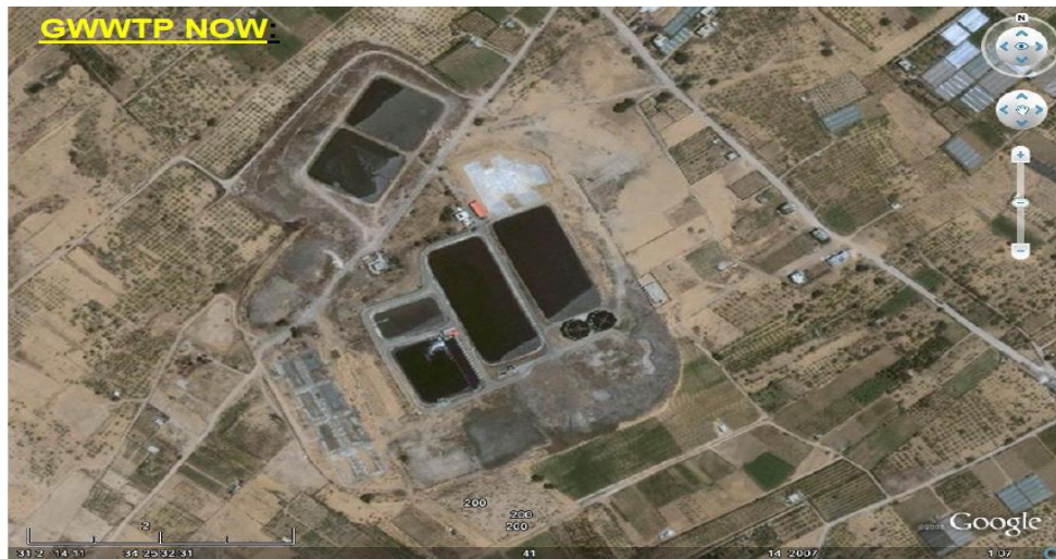
Figure 3.1: Gaza Wastewater Treatment plant (GWWTTP)
