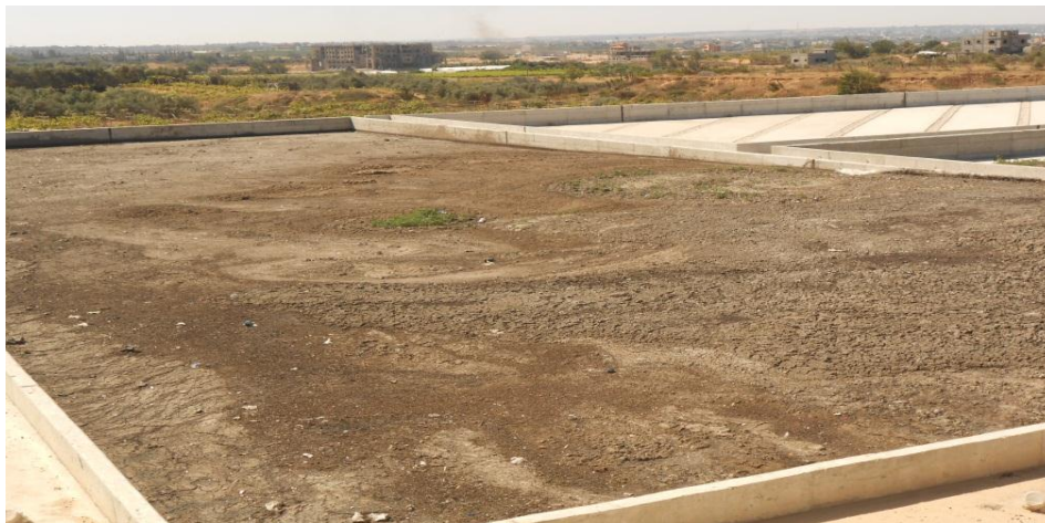
Figure 3.2: The drying beds of the sludge at GWWTTP
